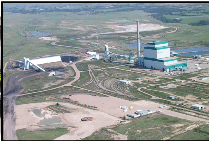
Shand Power Plant, Estevan, Saskatchewan
